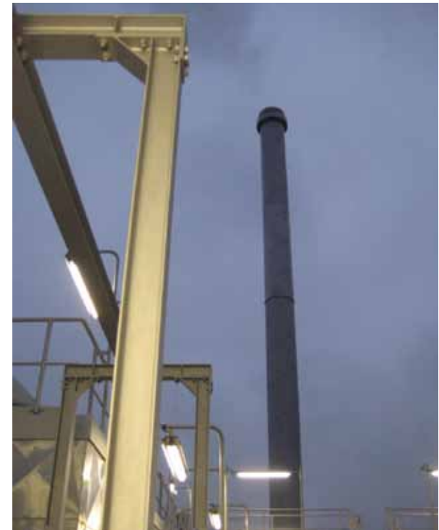
A view of the 80 meter tall stack.
